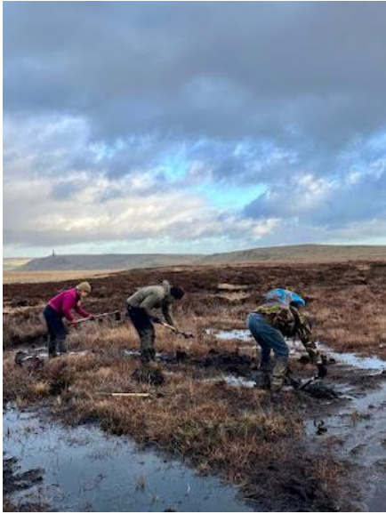
Drainage on Langfield Common.
