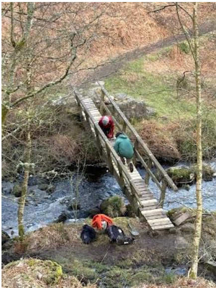
Bridge repair at Blake Dean.
