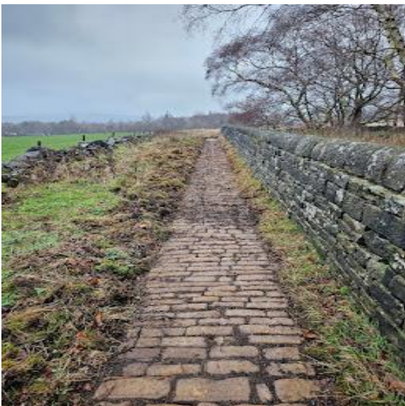
Path clearance at Longley Lane, Ryburn.
