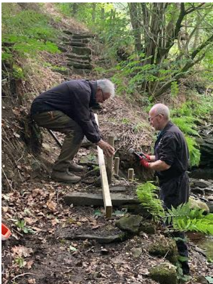
Revetment in Luddenden.
