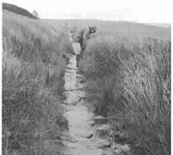
Drainage work on a causey path at Whirlaw.
